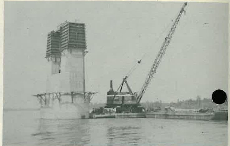
Here is pier No. 11 on the main river.
