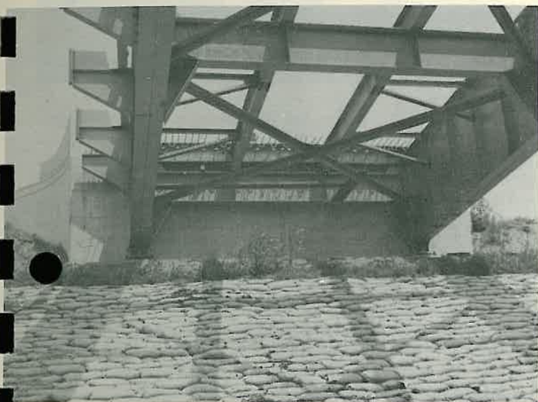
Here is the east approach showing concrete sand rip-rap on slopes.
